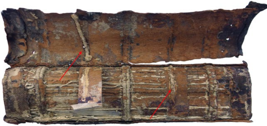
Fig. 8. Three double sewing supports and two false halfbands visible in the spine of a damaged book (VUL II 2232/1–13).
